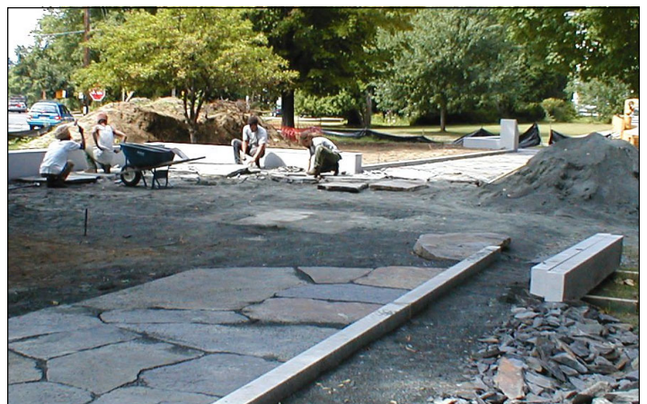
Stone Creations owner Paul Forth and staff, shown laying paving stones at the Sojourner Truth Memorial Statue site.
